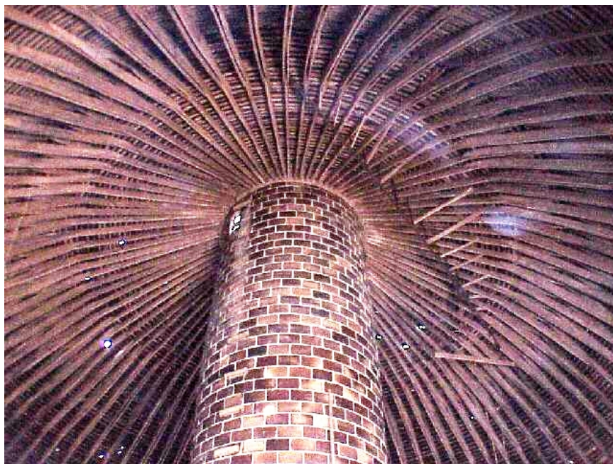
View of the interior silo/roof
